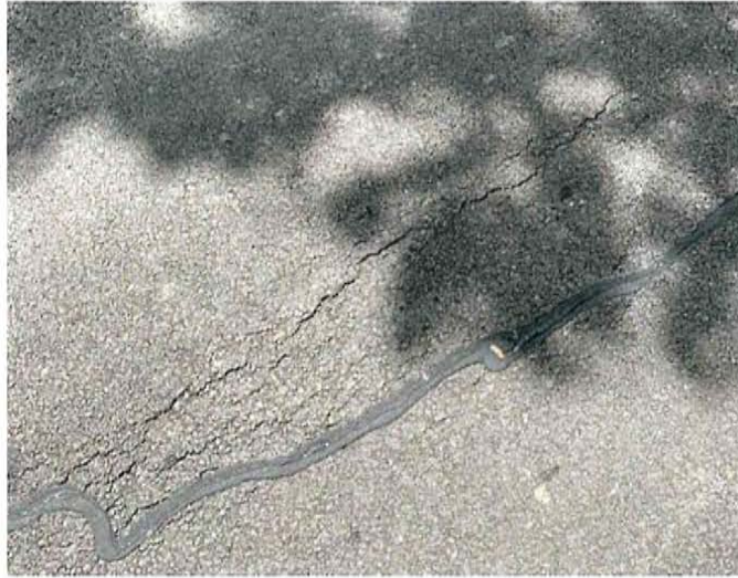
Image No. 2: Sealed crack and new developing cracks near southern edge of Ridgeway Drive, Blue Ridge, Texas, August 23, 2019.
