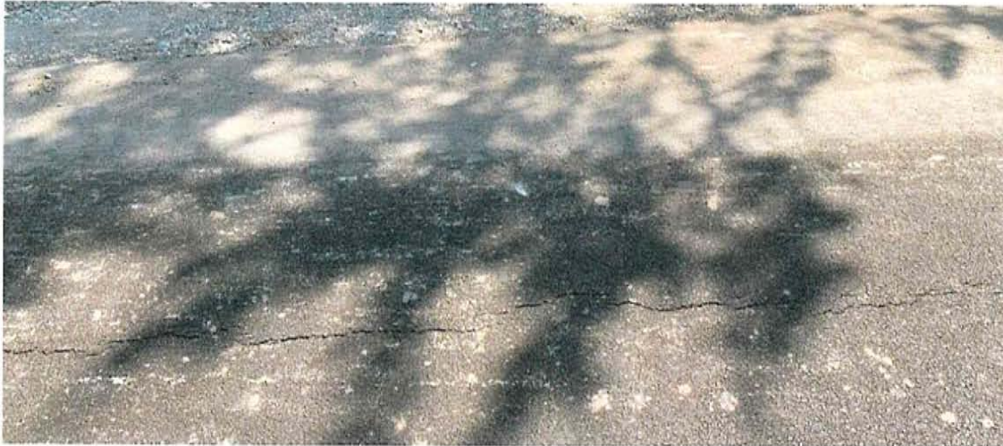
Image No. 1: Longitudinal cracking near southern edge of Ridgeway Drive, Blue Ridge, Texas, July 30, 2019.
