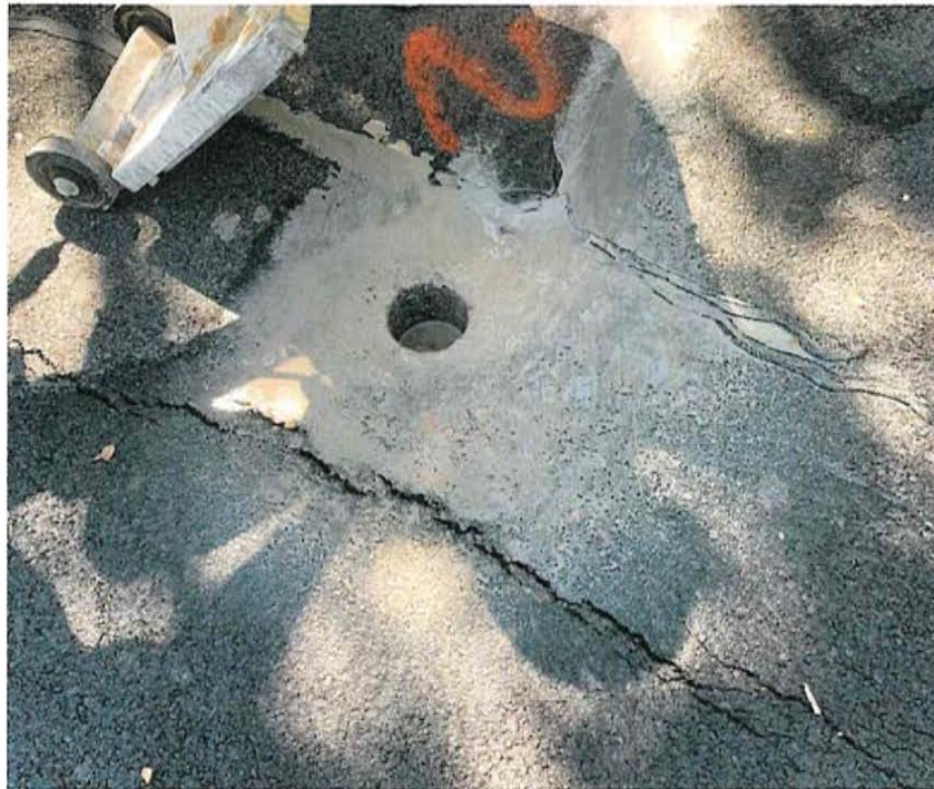
Image No. 3: Sealed crack and new developing cracks near southern edge of Ridgeway Drive, adjacent to Boring No. 2, Blue Ridge, Texas, September 17, 2019.
